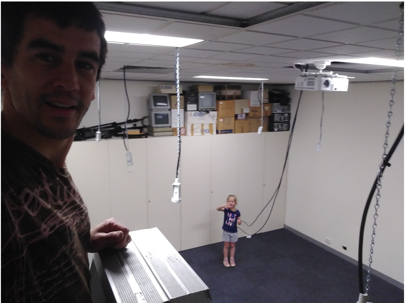
Stephen and his tech apprentice daughter relocating some AV cables
